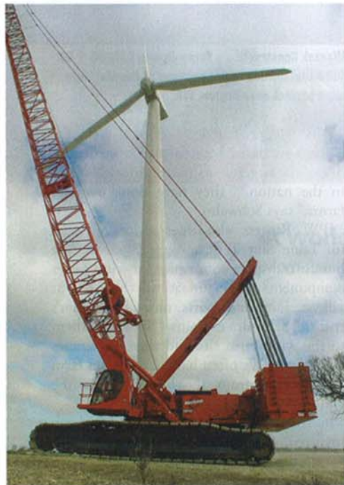
JPW's Manitowoc 16000 at a wind farm in Sweetwater, TX
