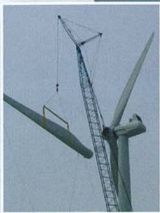
JPW Riggers handles a blade change at a wind farm in Maple Ridge, NY
