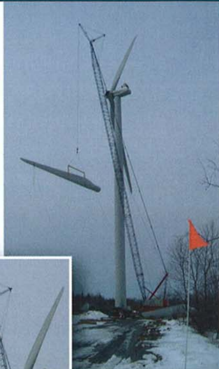
JPW Riggers handles a blade change at a wind farm in Maple Ridge, NY
